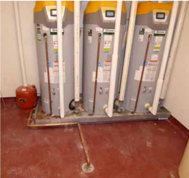
*Water heater drain routed to floor drain in center rather than one along perimeter*
