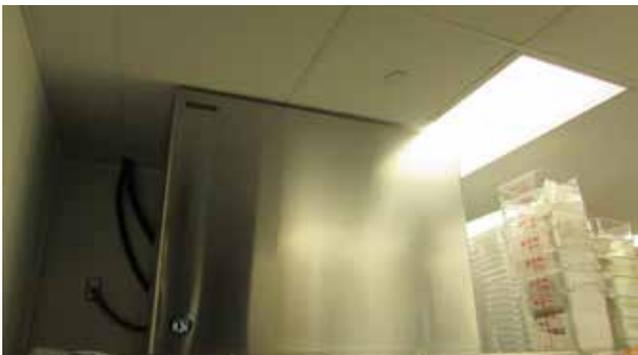
*Ice maker production reduced due to no ventilation above unit. Unit obstructs access to lighting fixture.*
