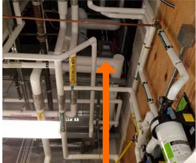
*Air handling unit with no access for service, which results from of lack of site supervision during construction*
