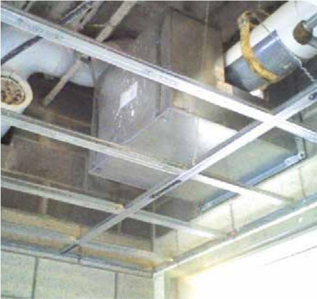
*Roof drain leaders routed through outside air intake duct*
