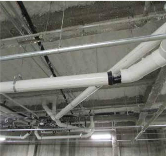
*Plastic drain pipe used for beverage conduit*
