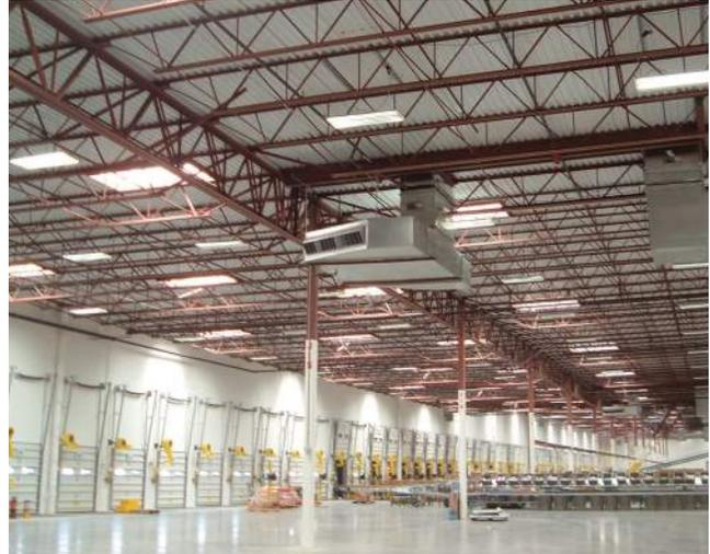
Areas that are required to have multi-level controls shall be controlled by “partial-on” occupancy sensors (only 50-70% of the lights shall turn on) or vacancy sensors (manual-on only).
